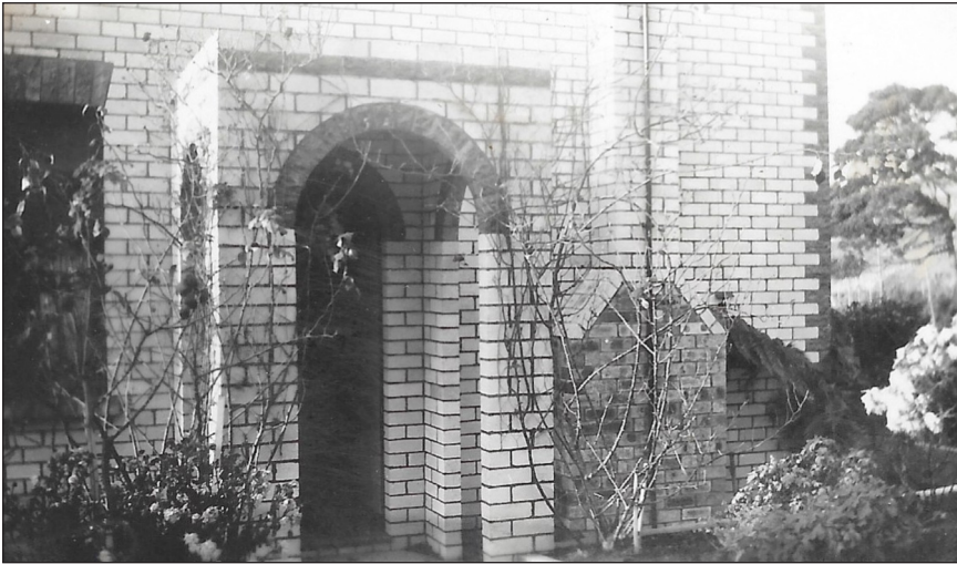
John's last brickwork in Huntly
