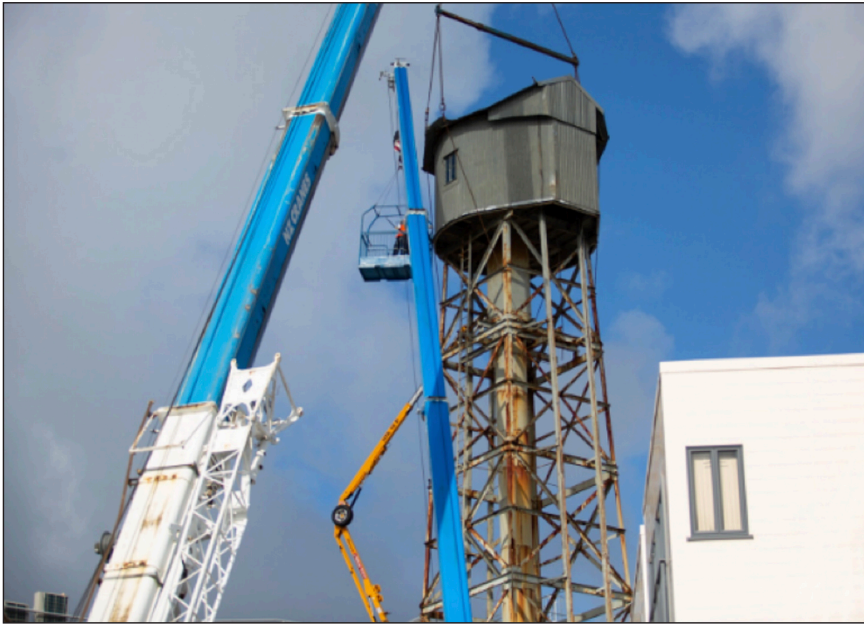
The shot tower during demolition in February 2023
