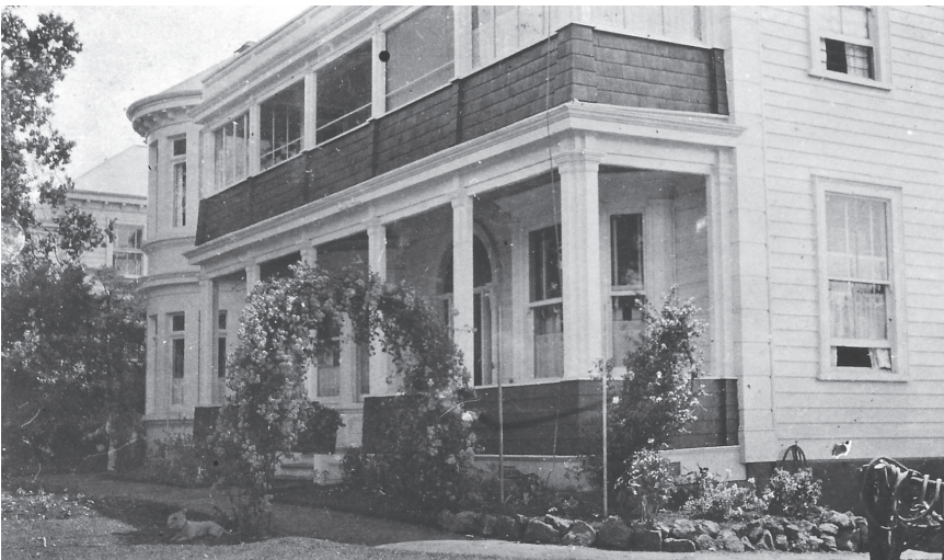
Fig.2) The front of the house has been altered from the more elaborate Victorian style verandah (of the previous photo) and clearly shows the 1908 addition of the double height bay window (left).
