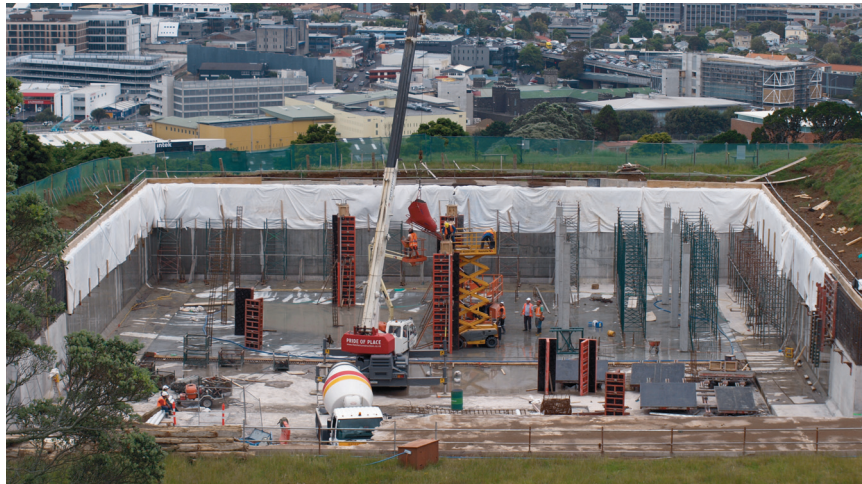
Mt Eden Reservoir rebuild
