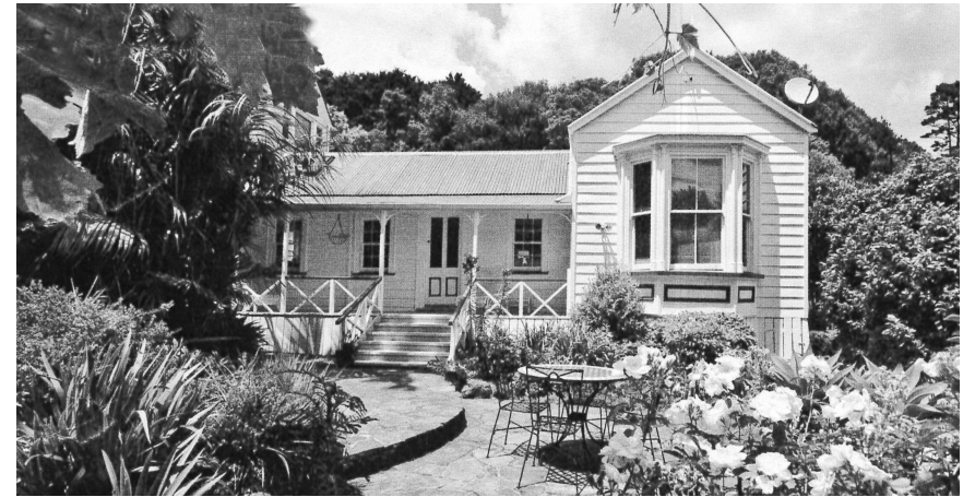
This building, still standing at 17 Hillside Crescent South, housed the first privately-owned tearoom on the slopes of Mt Eden, not far below the kiosk. The original small cottage has been added to over the years.
