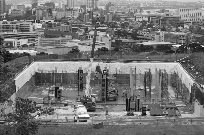
New reservoir under construction on Mt Eden
