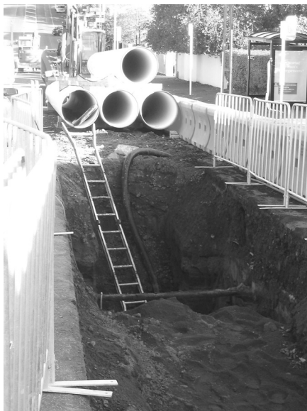
New water main being installed beneath Mt Eden Road
