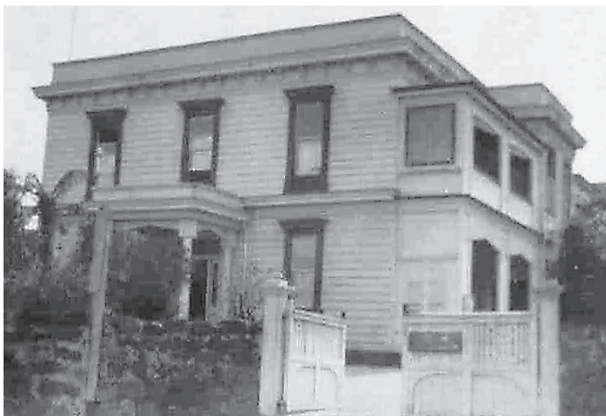
The original building as it was by 1915, looking from Stokes Road
