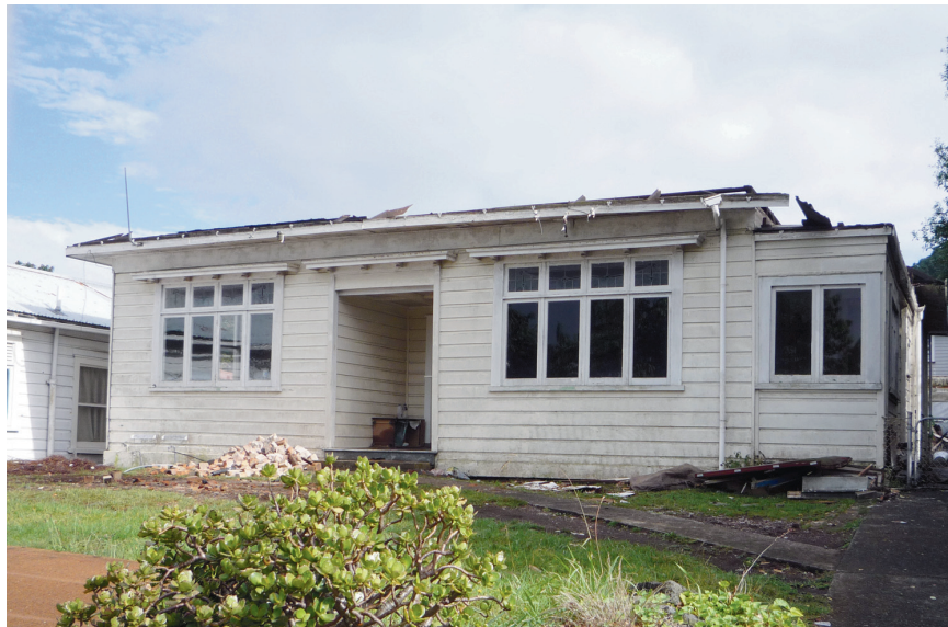
Demolition underway—the roof off early, January 2011
