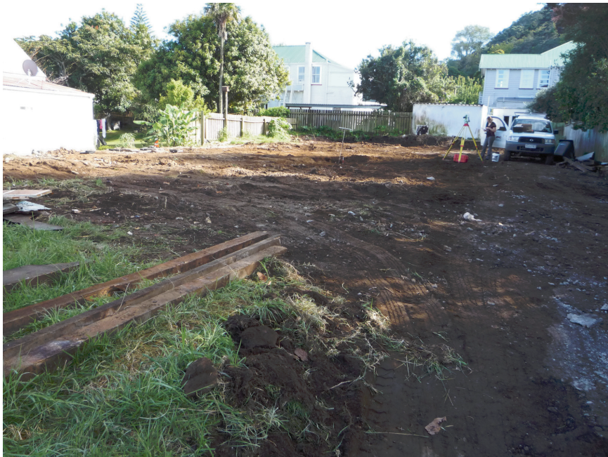
The site cleared ready for the dig, March 2011
