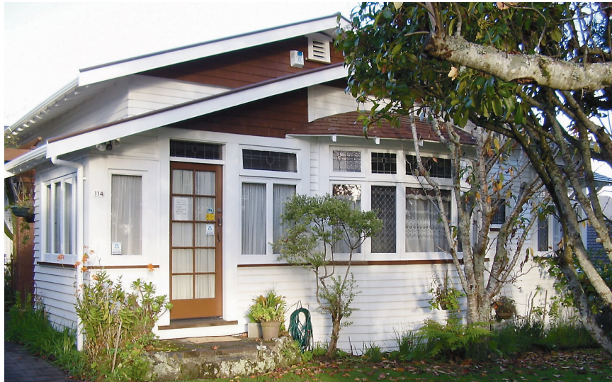
The alteration to the front to make the fourth bedroom
