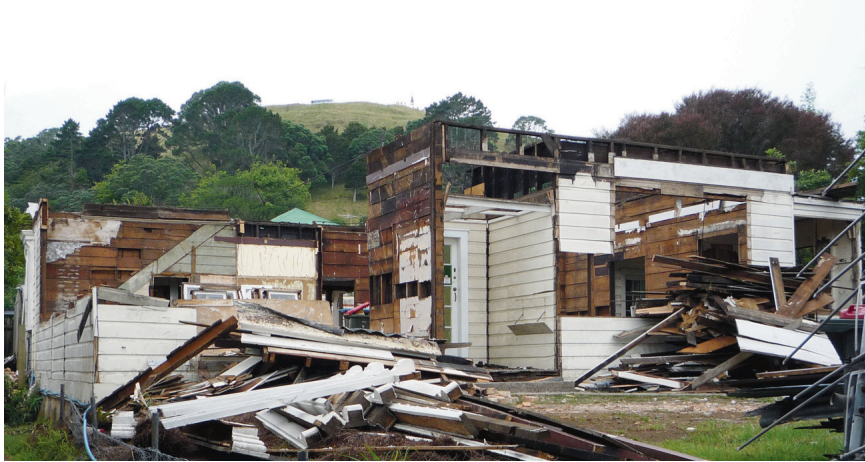
The original staircase and other construction details, mid January 2011
