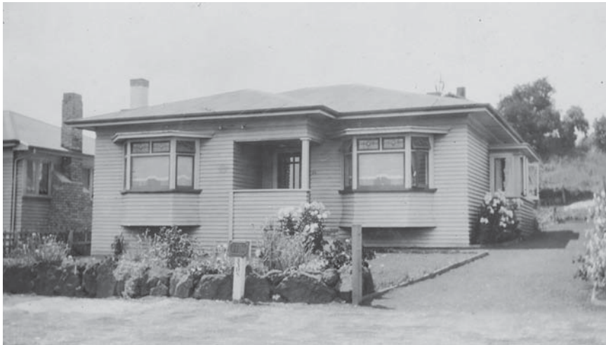
21 Gorrie Avenue. A simpler style of bungalow built in 1928 and occupied by the author of this article. Leadlight glass features on the fanlights, and the sunporch has been enclosed to provide an extra room. A front rockery used up many of the volcanic stones lying about.
