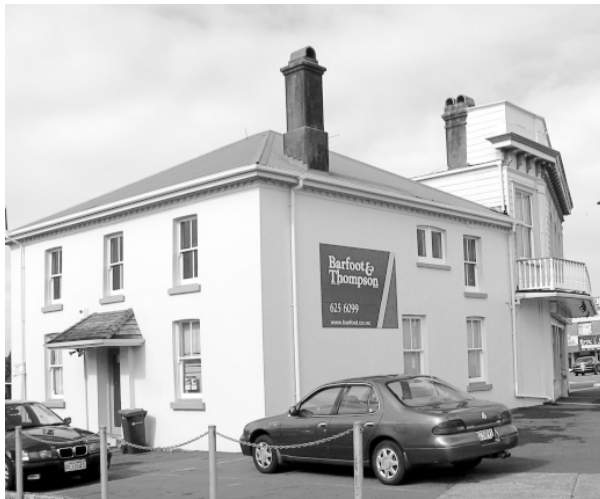
Rear of Royal Oak Hotel, 2004, showing original brick building.
