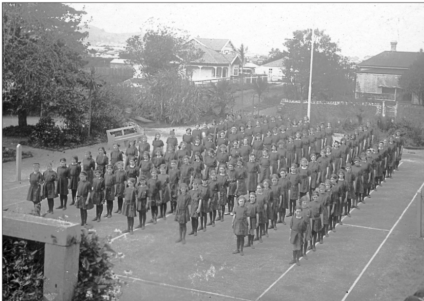
Pupils assembled on the tennis court on the western side of the main building.
