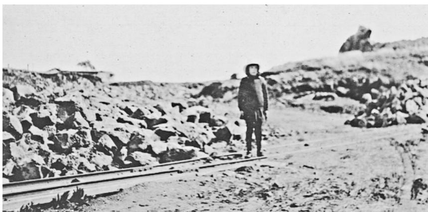
The site of Melville Park before development. Note the rails for wagons which were used to remove rock.
